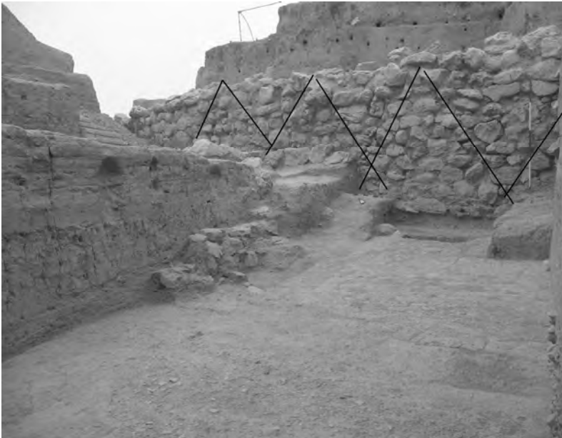
Fig. 11 J1. Revetment wall showing triangular pattern in unit J1 (Photo D. Mustafa)
