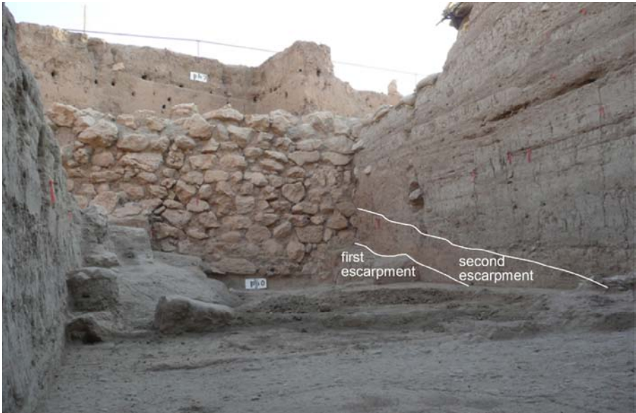
Fig. 5. Detail of revetment wall in J1
