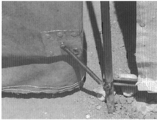
Ill. 8 – Detail of spring holding in place the lower corner of the protective tarp. Design of Sabah Kassem (photo G. Buccellati V17d9201).
