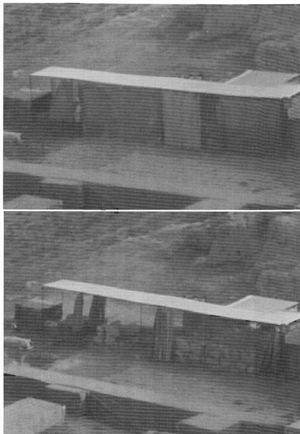
Ill. 6 – The new system of wall covering in AK, room B1 a. with tarps drawn shut (photo D. Mustafa V17d9202) b. with tarps drawn open (photo D. Mustafa V17d9203) Looking north, with metal roof and different experimental types of tarps sliding horizontally.
