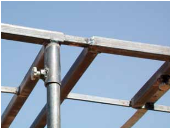
Figure 7. Detail of trellis, showing link among components.
