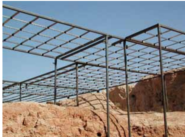
Figure 8. Detail of trellis, showing modularity of system.
