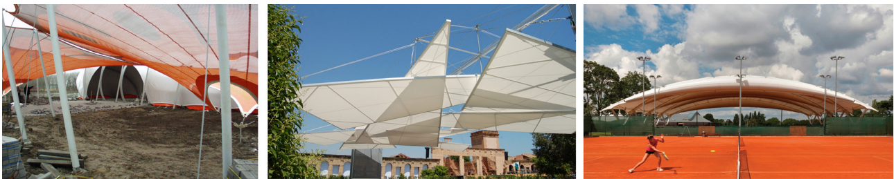
Fig. 2 - Textile sheltering examples, supported by (from left to right): a) tensile structures; b) a framed structures; c) removable pneumatic membrane arches (Source: www.tensinet.com ; www.tensoformsrl.com ; ww.vonsternberg.com )
