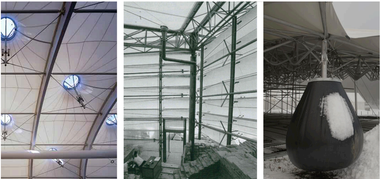
Fig. 4 - Functional textile details for solving the principal needs of archaeological shelters. From the left to the right: a) roof openings integrated into textile roof for indoor ventilation; b) vertical partitions and rainwater system; c) removable sandbags for tensioning the membrane (Source: www.canobbio.com ; Zanelli, 2015; www.tess.fr )
